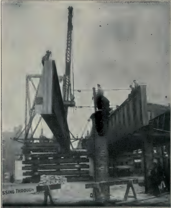
PLACING STEEL GIRDER OF RAILROAD BRIDGE
